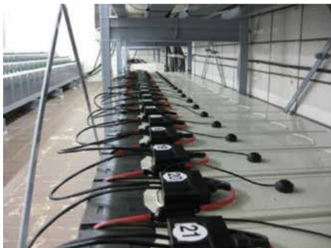
Civil Aviation Authority Installation, Europe
