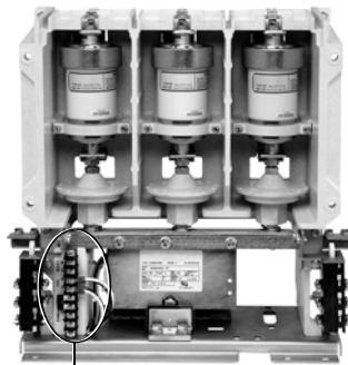
Control Terminal Strip
