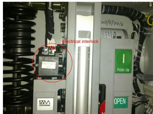
Fig. 5-12B: Mechanism Electromagnetic Interlock
