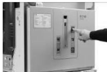
Fig. 5-4: Close manually
