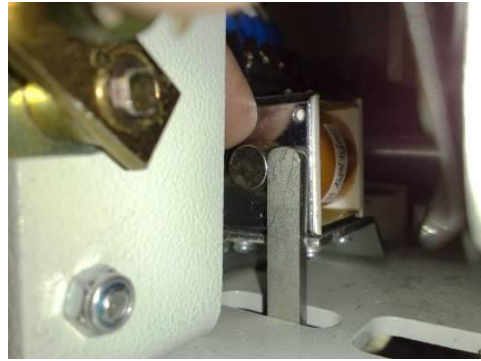
Fig. 5-11A: Cradle Electromagnetic Interlock
