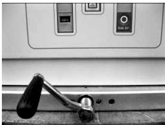
Fig. 5-8: Inserted racking Handle
